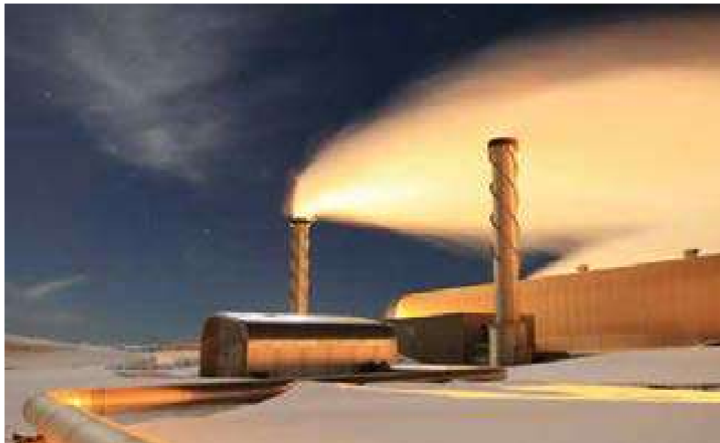
Geothermal Power Plant.
