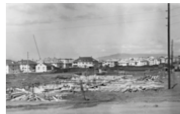
Hlíðar district in 1955. In the foreground we see the apartment block of Bogablið in construction. The farmhouse of Reykjahlíð can be seen on the left. (Photo: Borgarskipulag)
