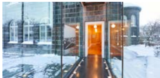
Old and new times, the corridor between Alþingishúsið and Skálinn. Kringlan can be seen on the right, built in 1908
