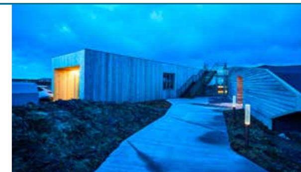
The new information center for Snæfellsjökull national park at Hellissandur was consecrated recently, beautiful building made by Arkis architects.
