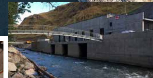
The Hydropower Station Exterior.
