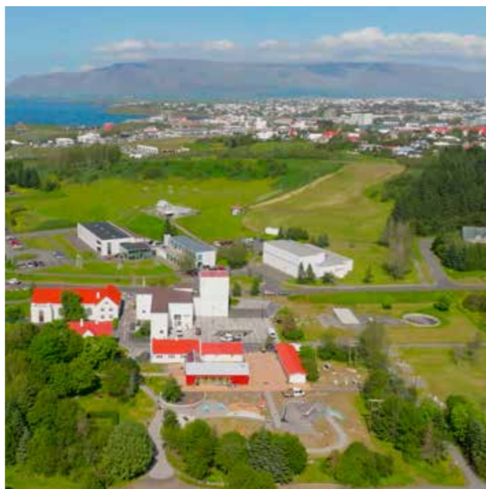
Once the beginning of electrification in Reykjavik, Ellidardalur Station is now a popular destination for locals and tourists alike.
