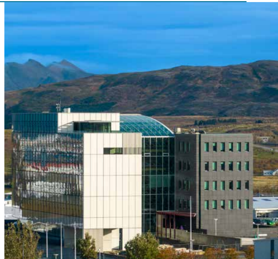
Reykjavík Energy Headquarters, and a future hub for energy startups and innovators.
